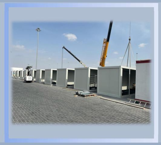
Bottom and Top chasis shipped as completed, only walls, doors and windows are needed to be installed at site.
